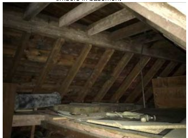
Photo 18. General view of roof void accessed near 1 st Floor Female Toilet
