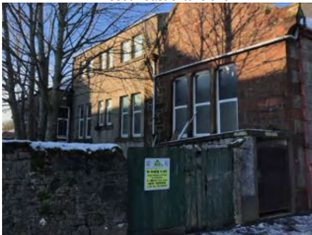
Photo 15. General of south-east elevations
