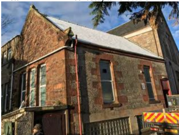
Photo 9. South-east corner elevations
