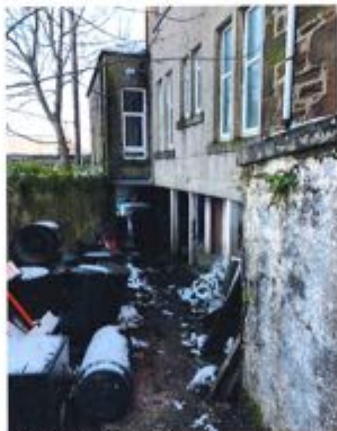
Southeast elevation (undercroft)
